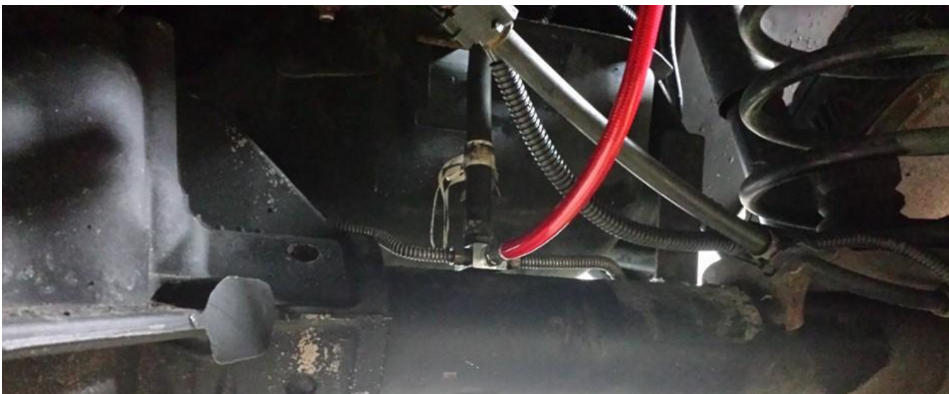
Axle-end brake line distribution block with vent hose hooked up
