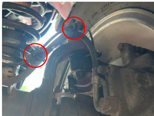
Old brake-line clips to be removed
