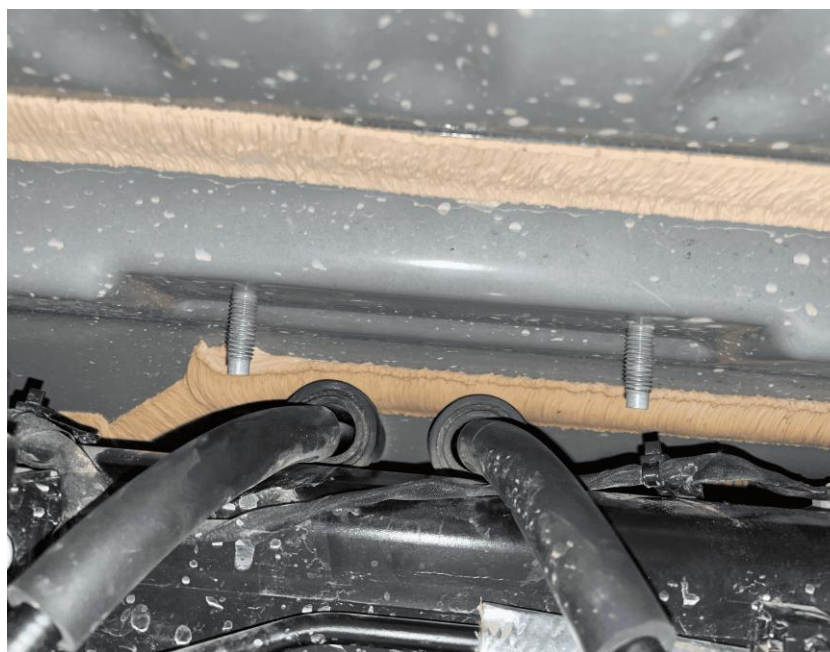
Figure 24: Emergency cable bracket removed
