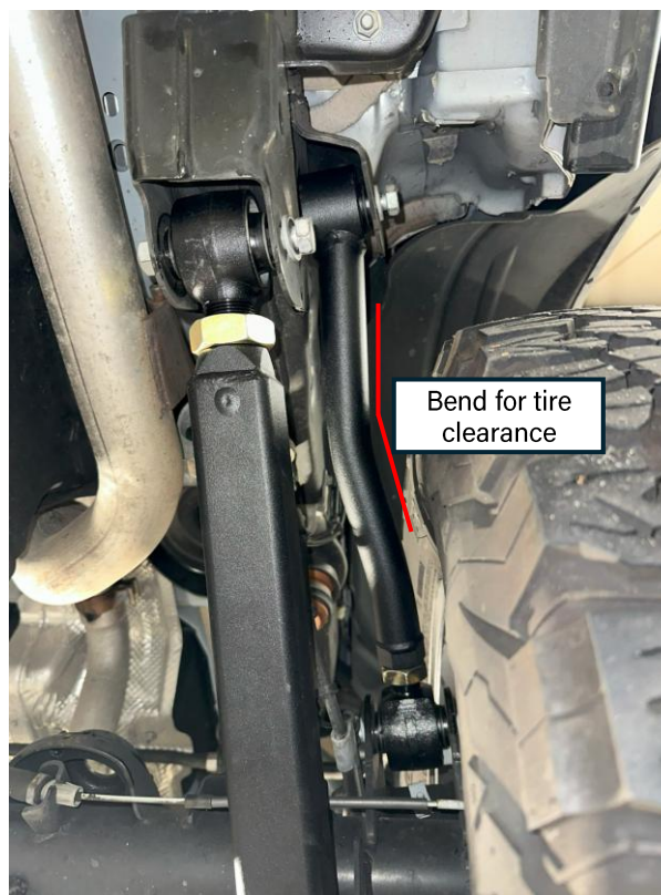
Figure 28: New driver-side control arms installed with original hardware
