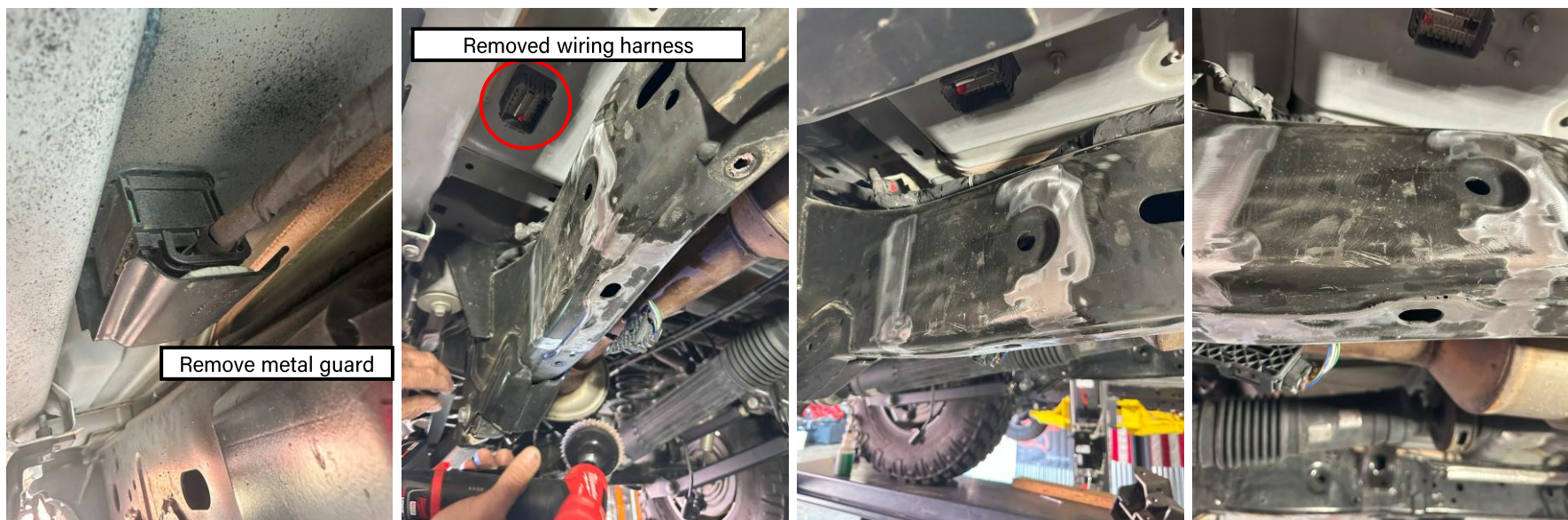
Figure 44: Frame rails prepped for bracket positioning
