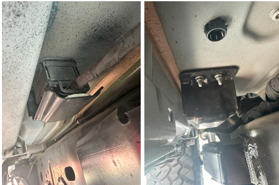
Figure 58: Wiring harness (both sides) reinstalled
